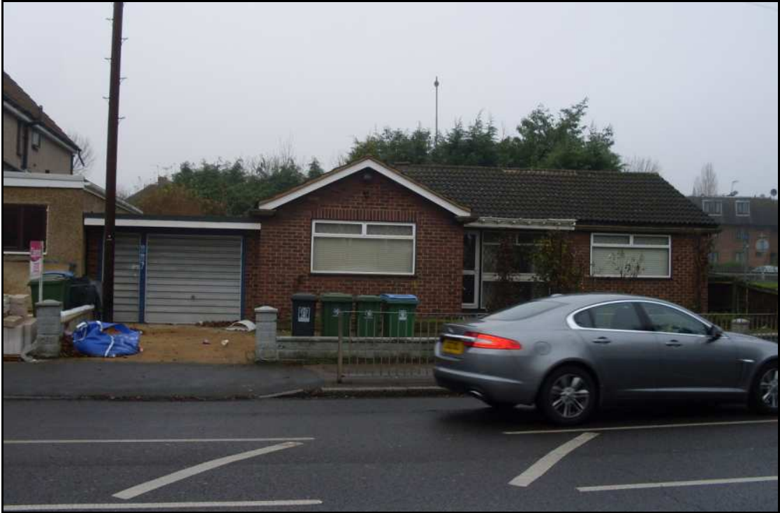
Front elevation of existing bungalow
